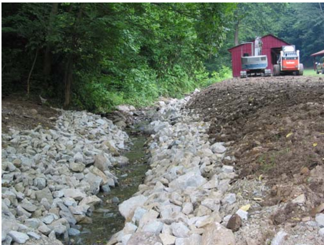
Banks have been regraded to a 1:1 slope. Boulders have been placed at the toe and stones above.
